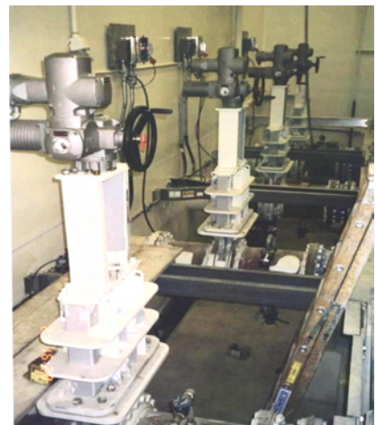
20" Fig 176 KGV with electric motors operators and handwheel override. Pictured here installed in a pumping station.
